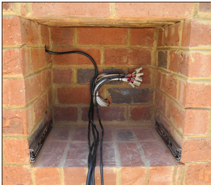
Rails Properly Mounted in Cavity
